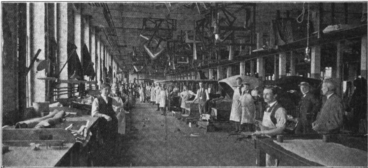
The trimming room, where the automobile body is received after the first three coats of paint have been applied. From here the body is returned to the painters for the completion of their work.
